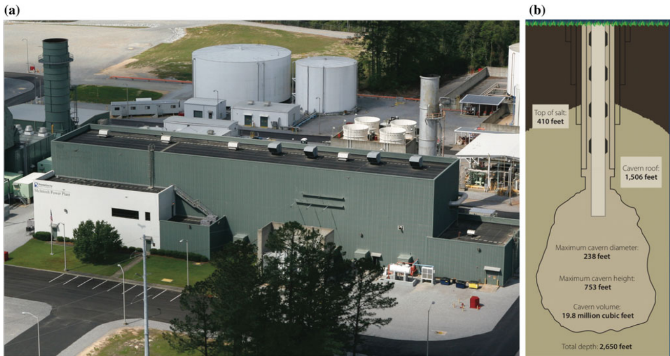
Fig. 7.3 a The PowerSouth energy cooperative McIntosh CAES power plant and b the pertinent salt cavern dimensions [2]
